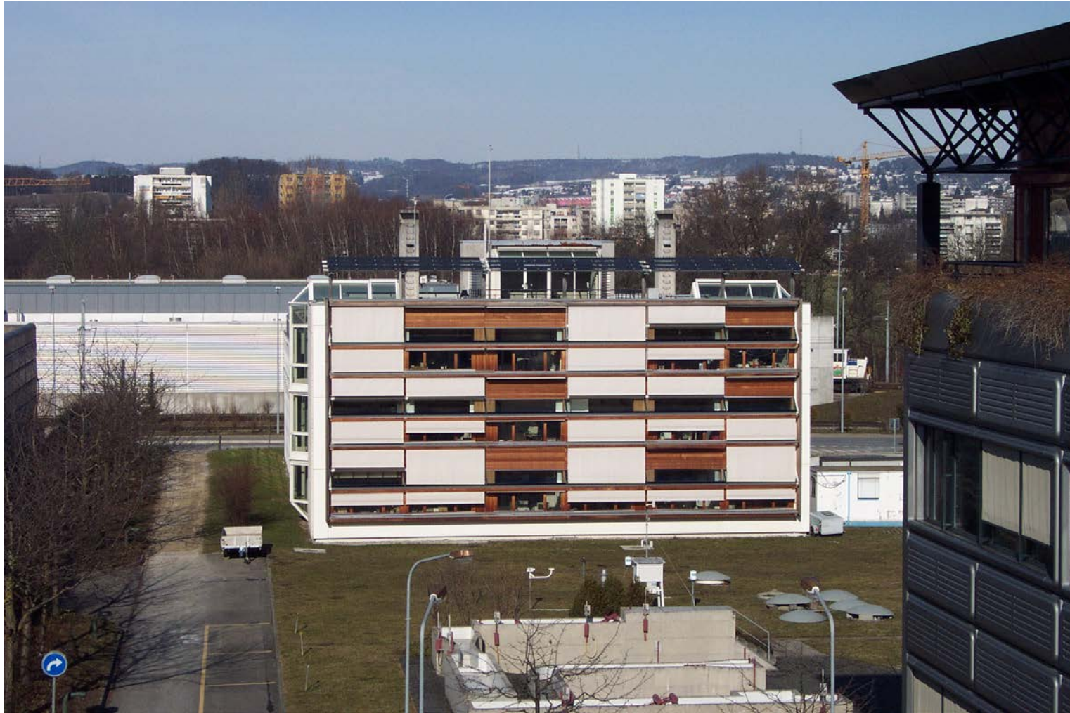
Project: LESO- BP (Solar Energy Research Institute)
